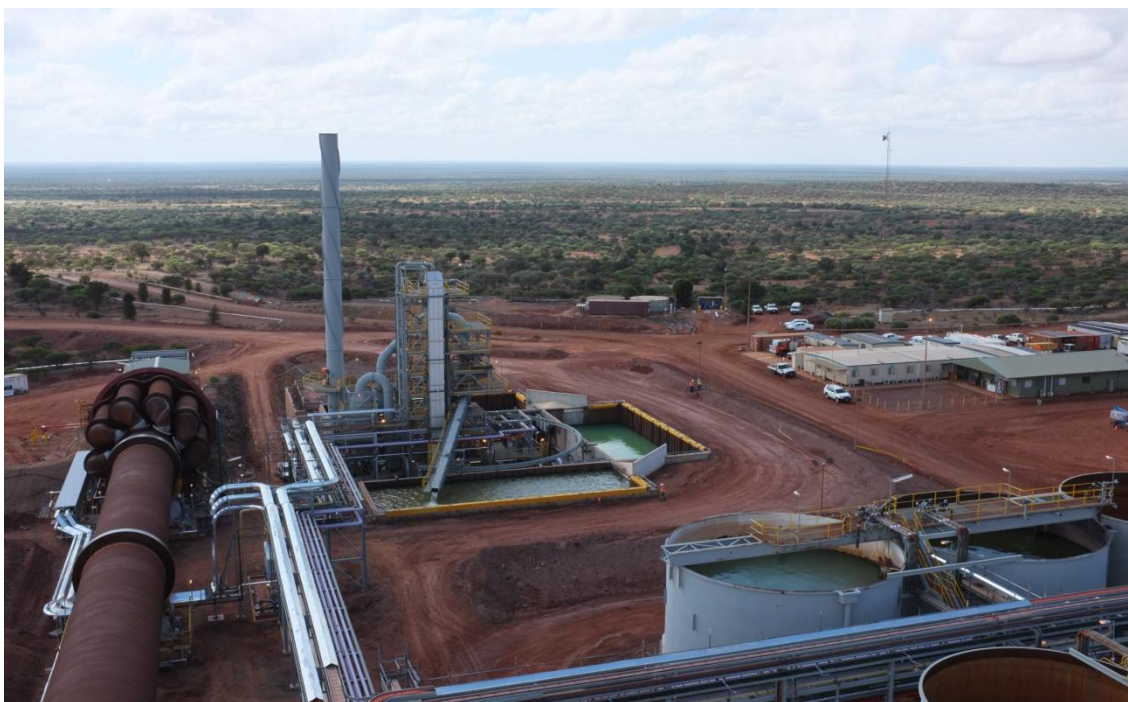
Kiln and leach vats undergoing wet commissioning
