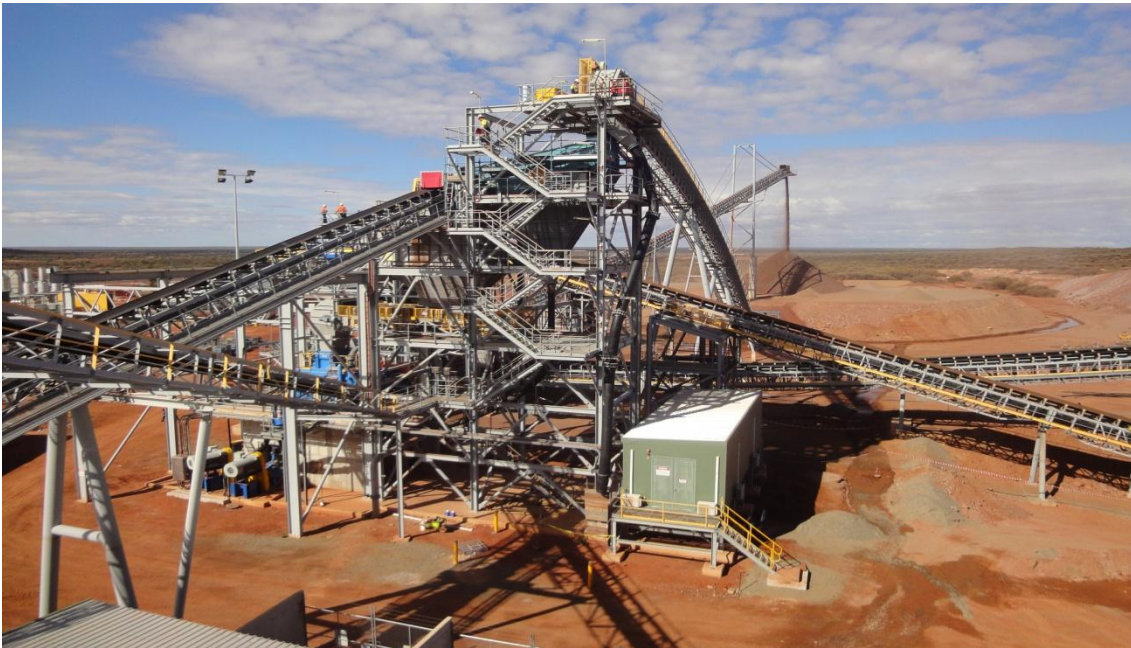
Building of the crushed ore stockpile
