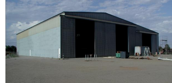
Port capacity secured at Berth 6
