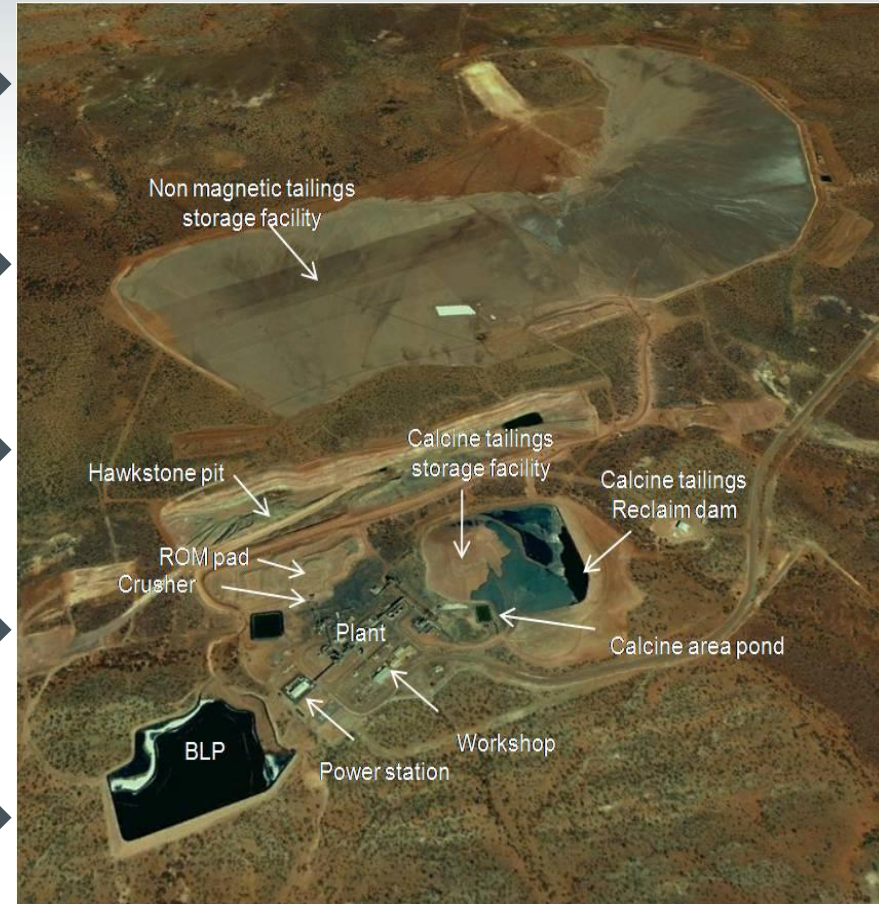
Aerial view of Windimurra mine and plant
