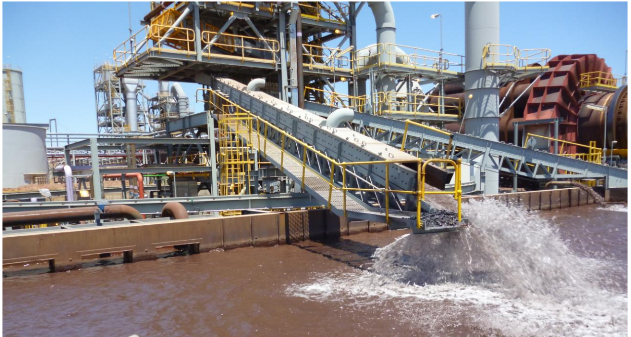
Roasted magnetite concentrate from the kiln undergoing leaching in the vats
